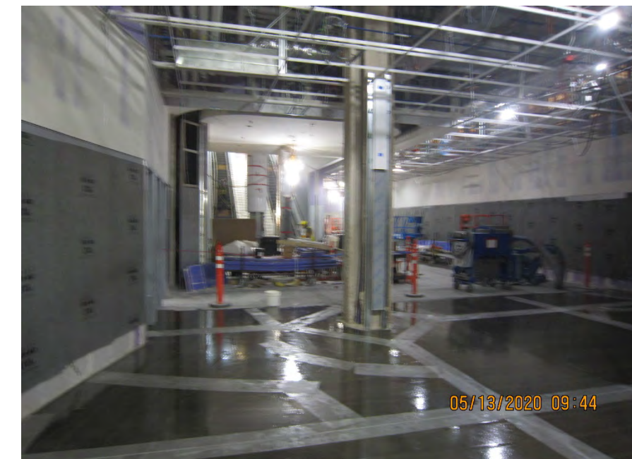
Basement: Terrazzo Prep at Bottom of C4 Grand Escalator
