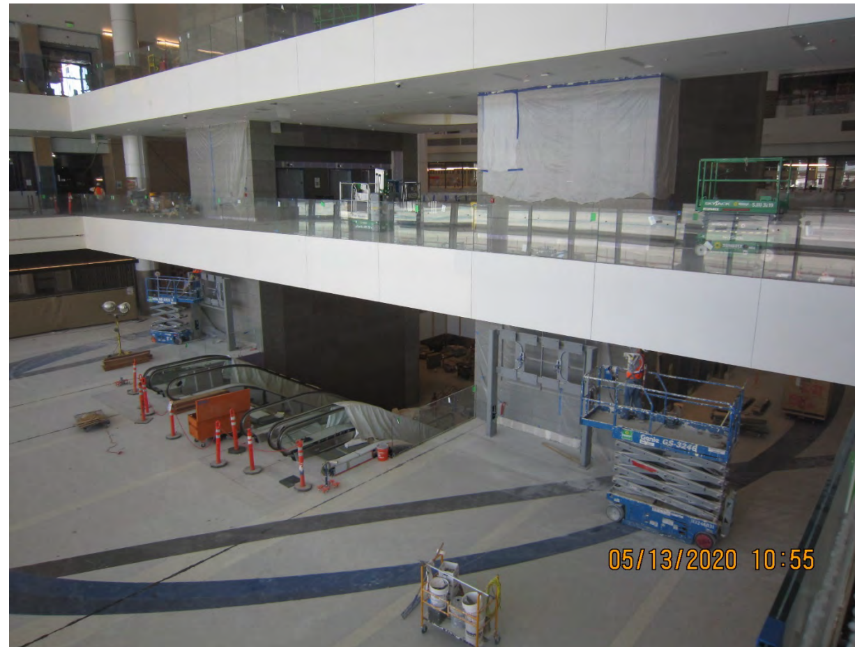
Gyp Ceiling Sanding Activities by PCI (Blue Lifts)
