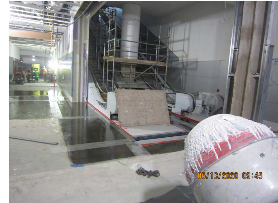
Basement: Terrazzo Prep at Bottom of C2 Grand Escalator
