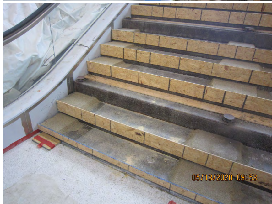
Sand Infill at Terrazzo Stair Treads at Core
