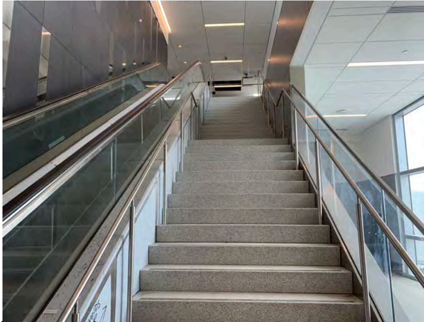
Terrazzo Stair and Glass Handrail Installed
