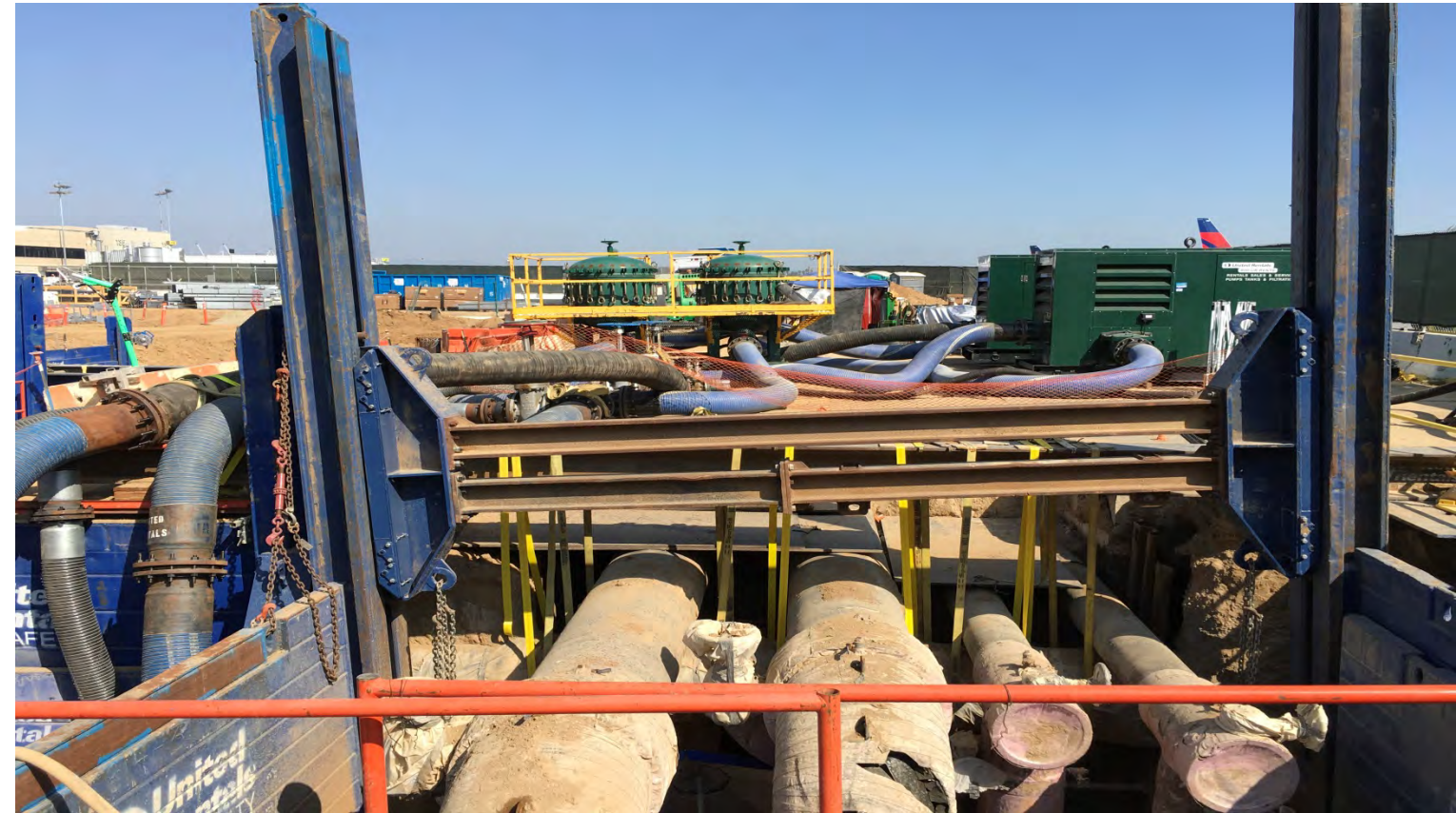
Area 3 – CHW Flushing System
