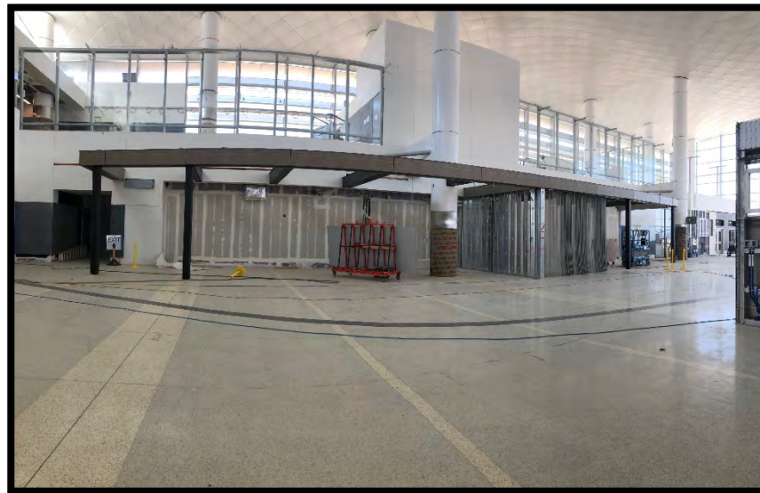
Neutral Framing at Concession Spaces N8 -finishes wrapping steel, security screen, and framing out at the concession spaces -most of MEP access has been coordinated at these spaces
