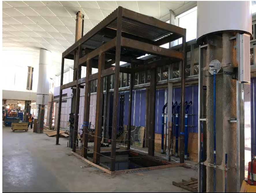
Service Elevator Extension
