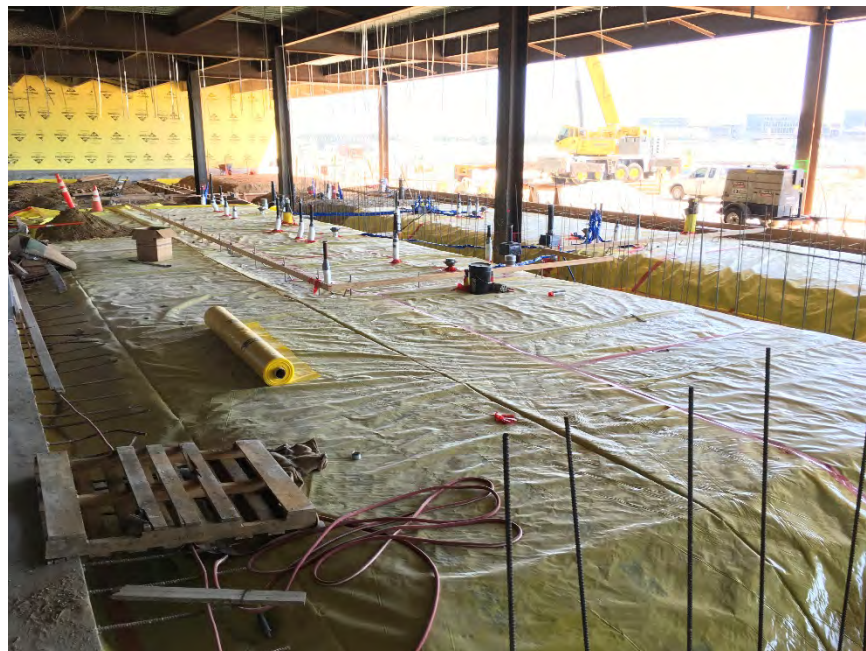
Slab On Grade Preparation at Core
