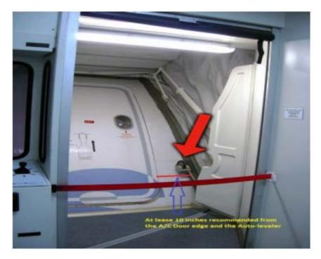
Another safety measure on the Bradley West PBB's is the safety show, which is a sensor that is placed between the aircraft door and the PBB floor.
