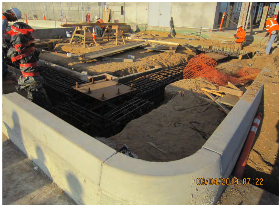
Group III: Foundation Work at N8-East Exit Sairs
