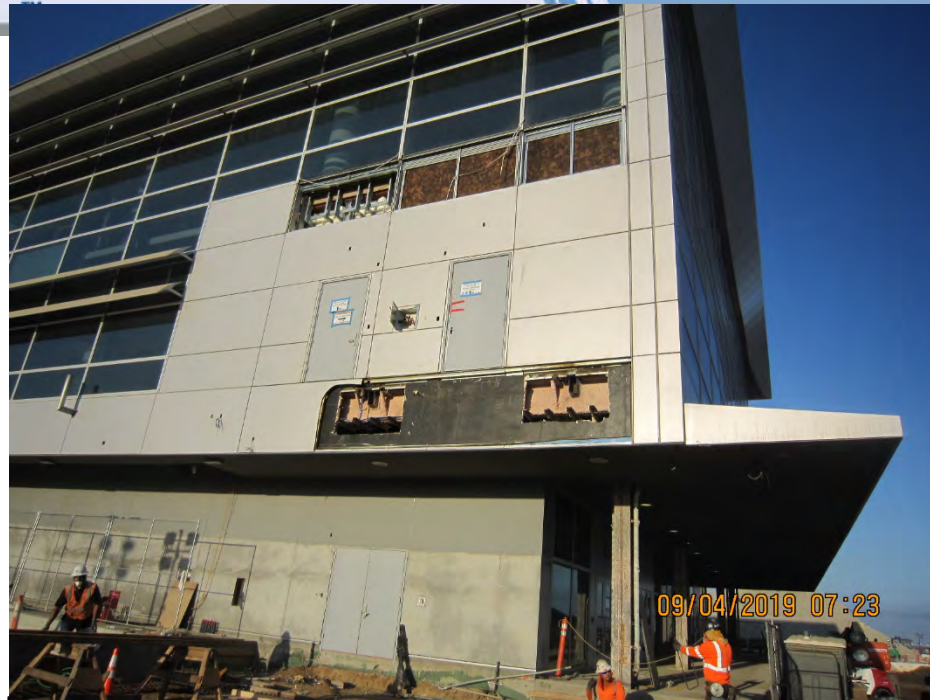
Group III: Demo of Metal Panels at Exit Stairs ( N8-East)
