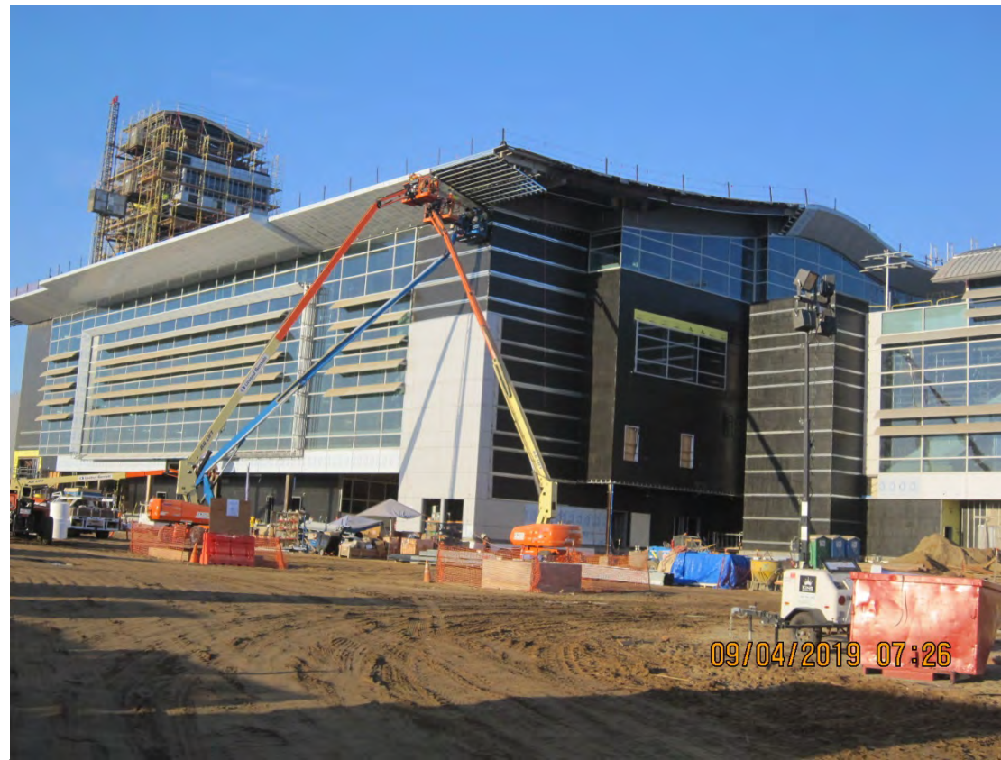
Metal Panel Installation Ongoing
