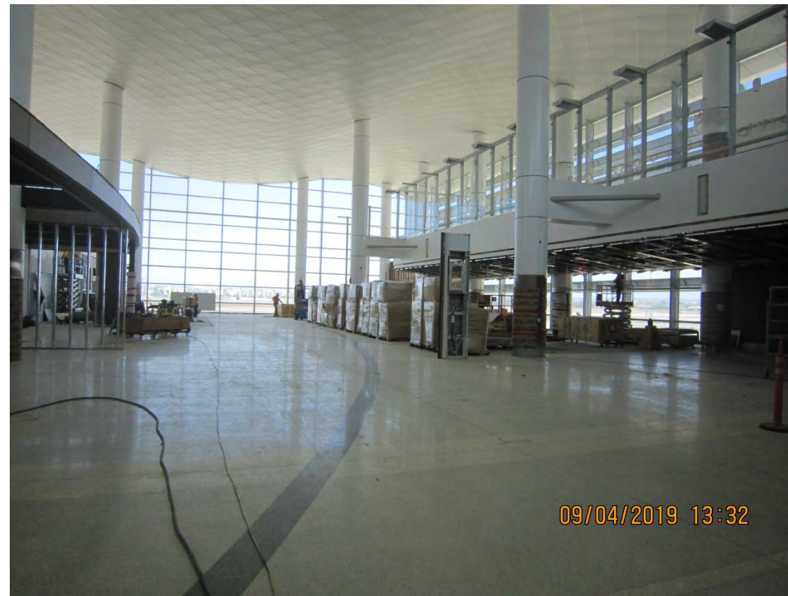
Conditioned Air Blowing at North end of Concourse. Getting Ready for Wood Ceiling Climatization
