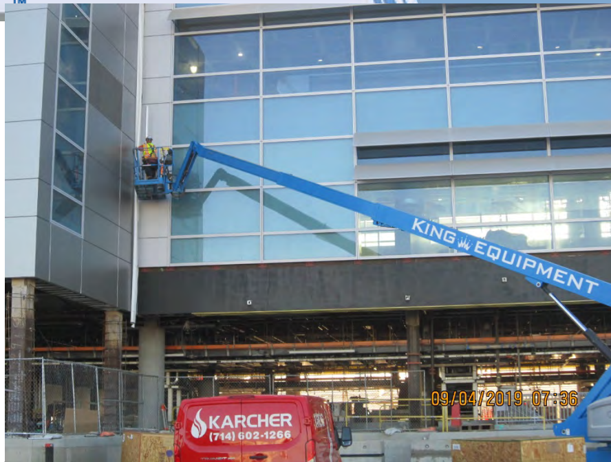
Expansion Joint Cover Installation at G204
