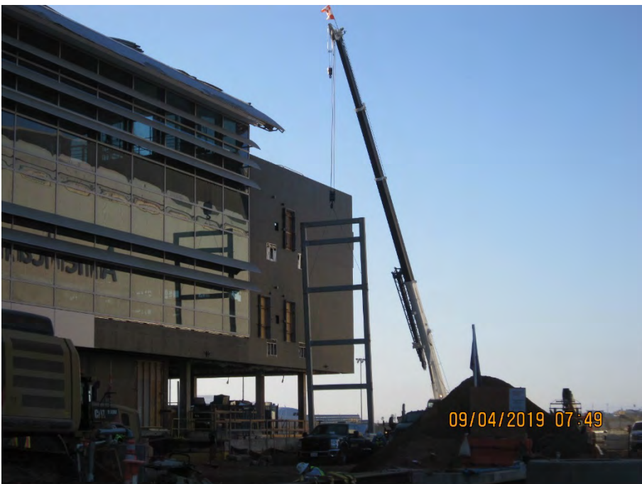
Exit Stair Installation at S2-West
