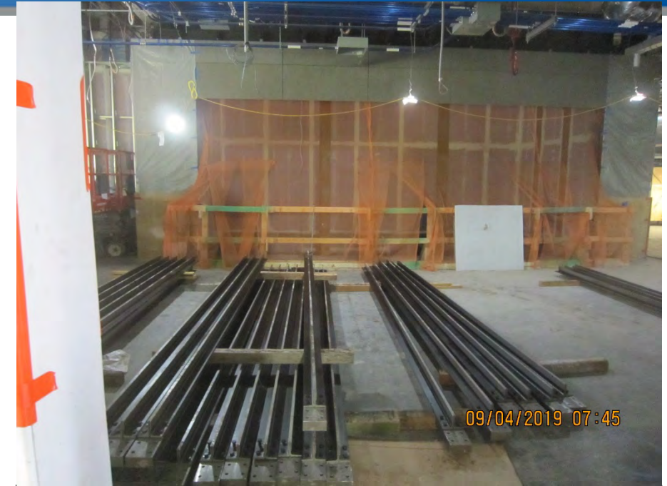
Elevator Guide Rails Installation at C2 - Apron
