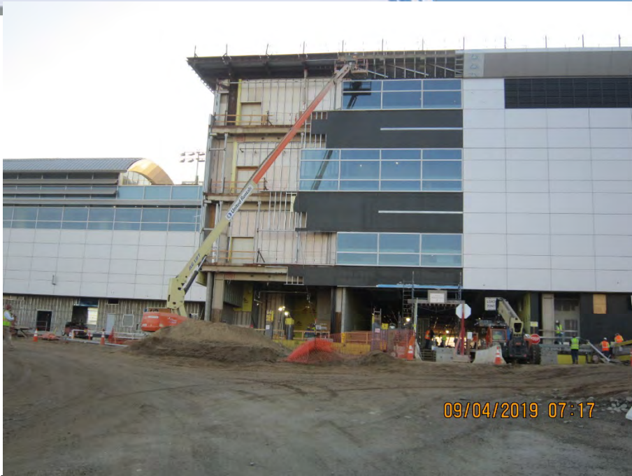
Man-lift Removed, Metal Panel Installation Proceeding
